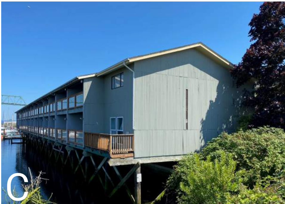
A: The original 56 unit built in 1972, showing large portions of gutters missing, decaying exposed structure, failing paint, and broken wood railings in many locations. B: Laundry and office built over the water with signs of moisture and decay. Unsatisfactory repairs to the foundation pilings with unsecured and irregular timber layout. C: West expansion showing missing siding, failing paint, and gutters that will cause moisture intrusion issues in the building envelope.
