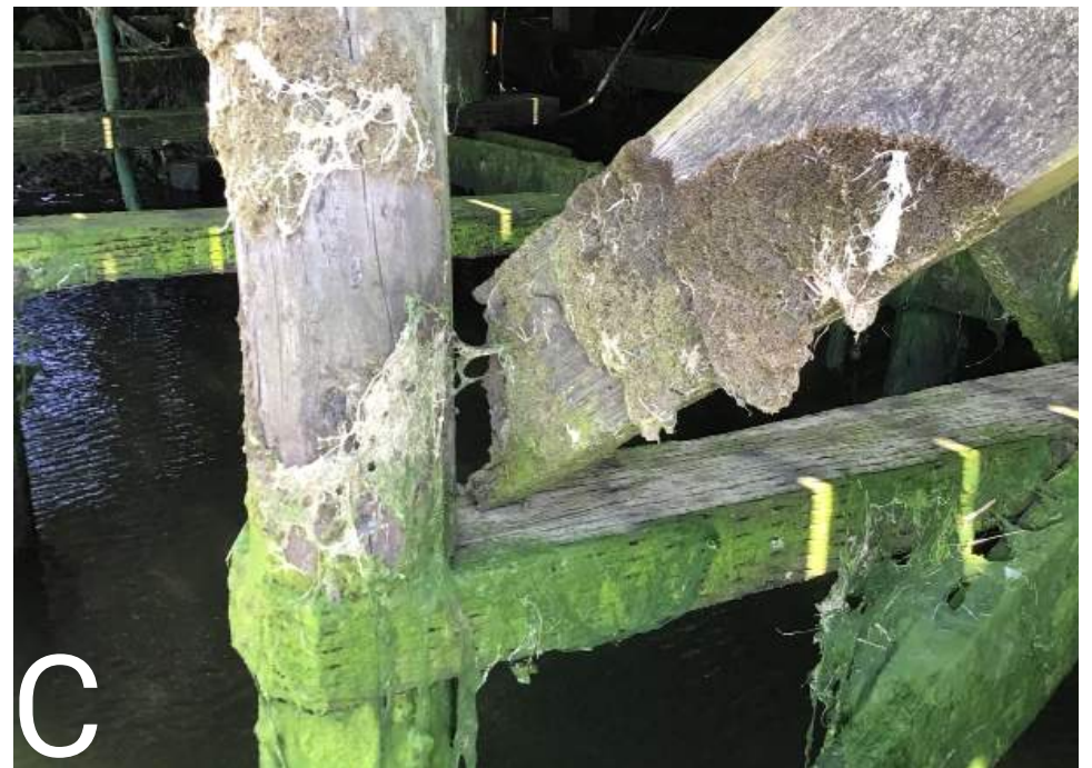
B: Decaying pier foundation under the Chinook building, some areas do not have continuous load paths to piles with minimal connections.
