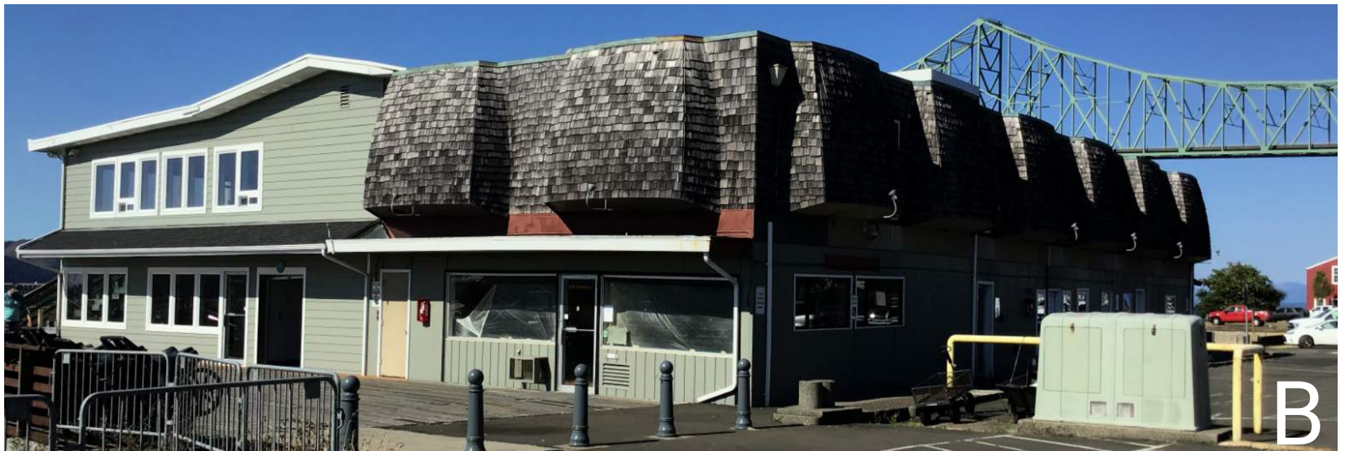
A: West elevation over the water with crane to unload fishing boats and equipment. B: South elevation (left) shows 1980s construction removed and rehabilitated, (right) is 1980s renovations showing deteriorated gutters, flashing, and drip edges that help to keep the building envelope dry.
